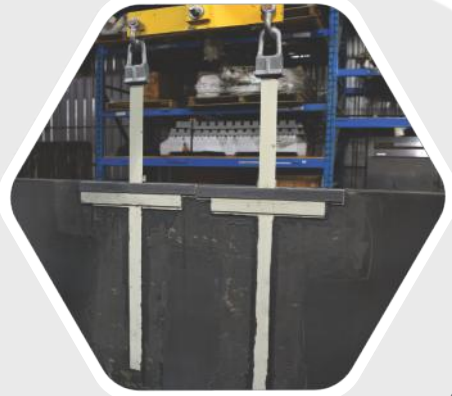
Anchoring Straps on the Inside Wall
